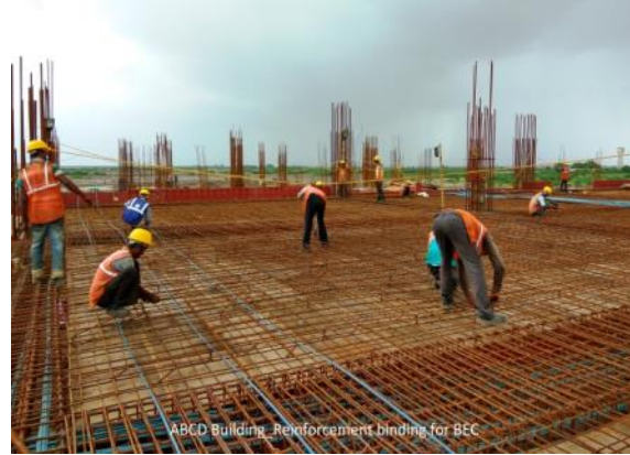
Reinforcement for BEC Slab
